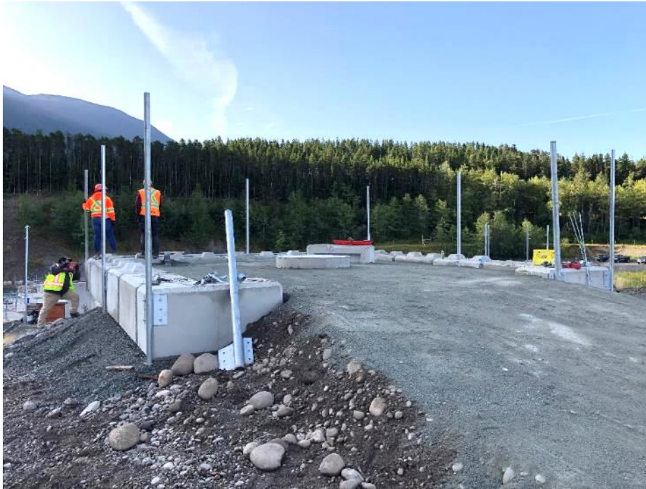
Photo 7 – Flare Pad Completed
