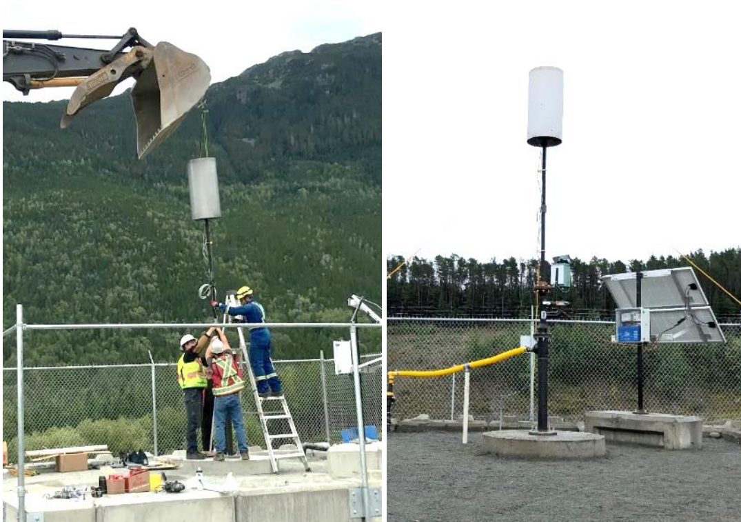
Photos 8 & 9 - RDKS and SHA Staff installing Solar Spark Flare
