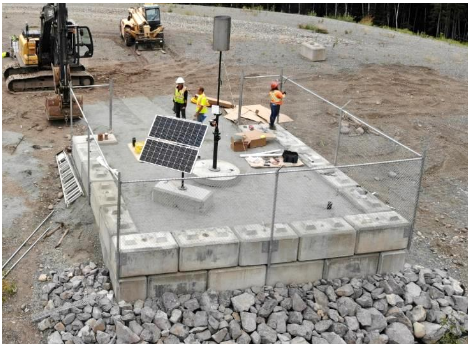
Photo 12 – Thornhill Flare During Installation (August 19, 2019)
