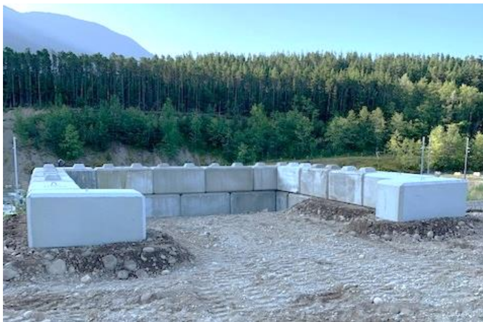
Photo 6 – Flare Pad Construction – Lock Block walls completed
