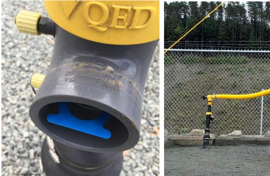
Photos 10 & 11 – Precision Wellhead and Orifice Plate
