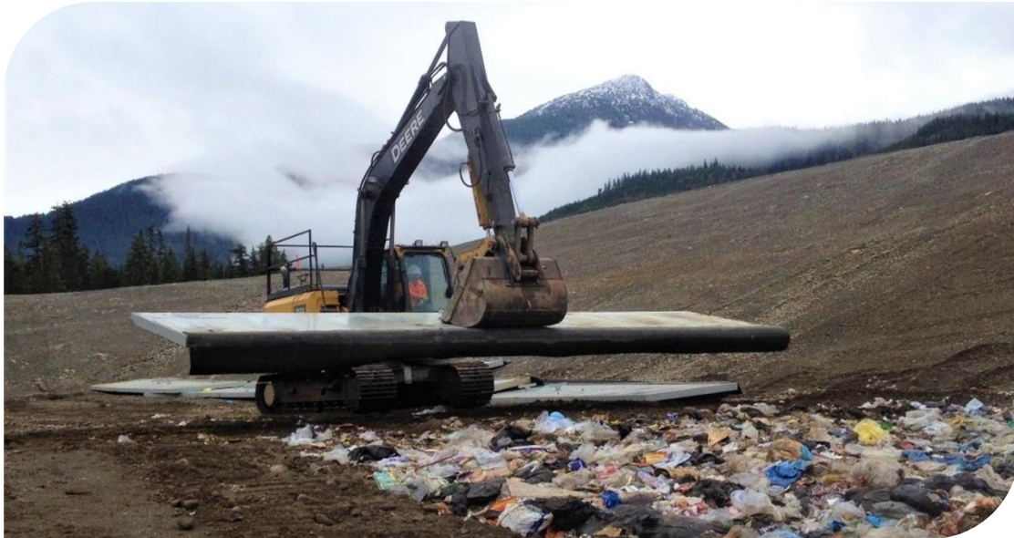
Figure 4 Placement of RIG plates as alternative daily cover at the landfill at Forceman Ridge WMF.
