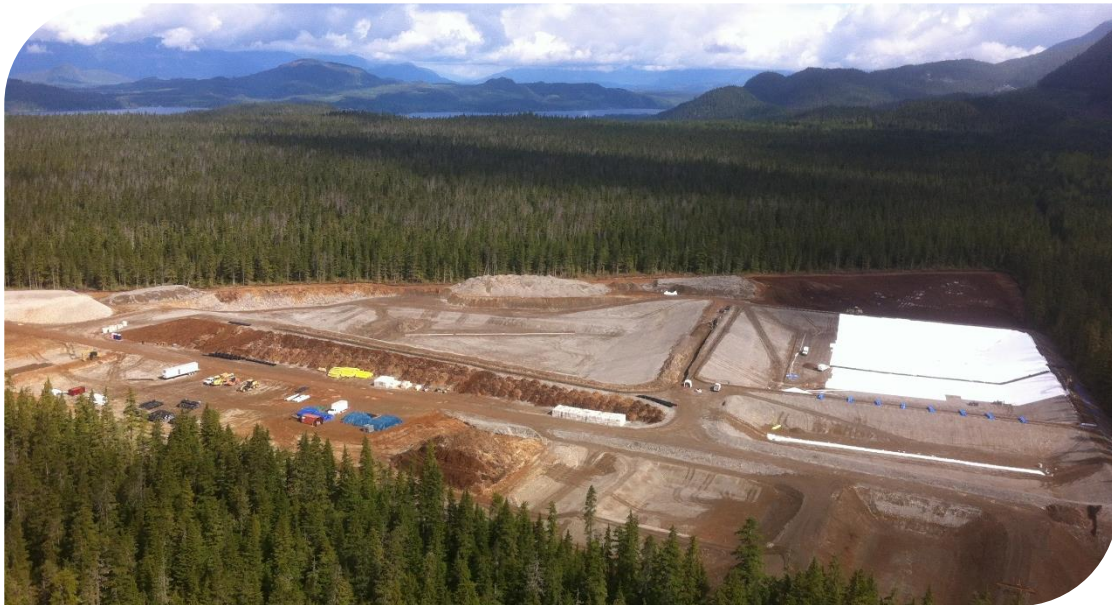
Figure 3 Forceman Ridge WMF under construction.
