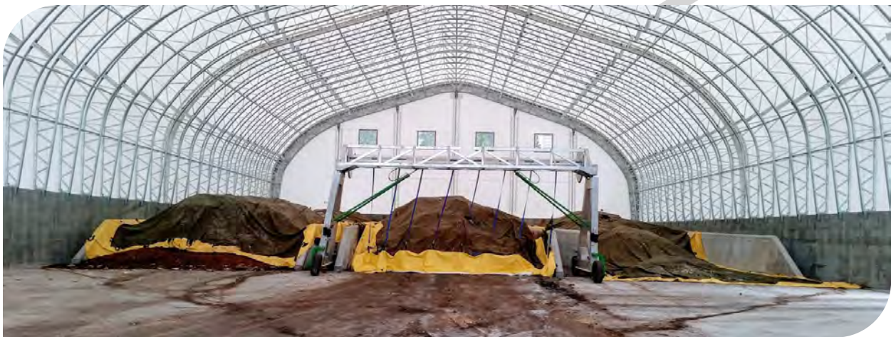
Figure 13: Composting facility at Forceman Ridge Waste Management Facility.
