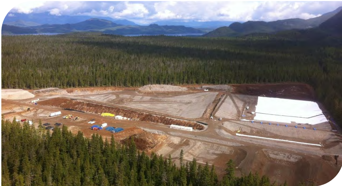
Figure 3 Forceman Ridge WMF under construction.
