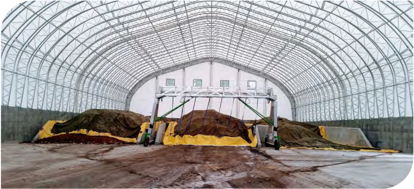
Figure 3 Composting facility at Forceman Ridge Waste Management Facility.
