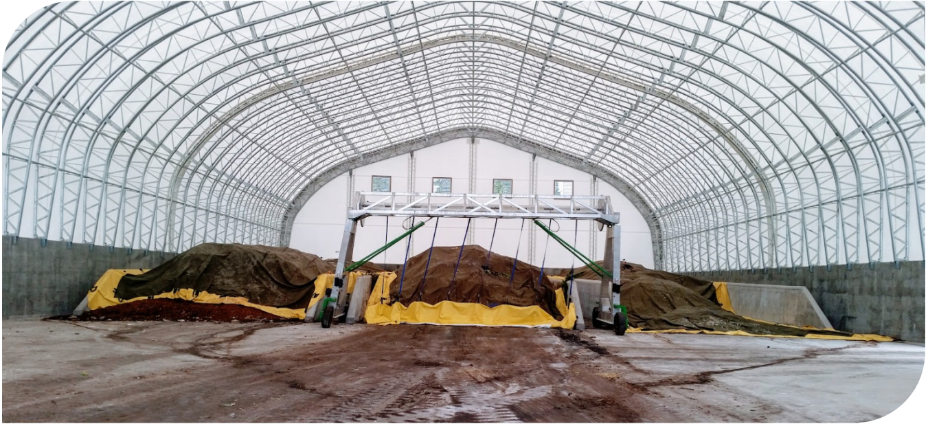
Figure 7 Composting facility at Forceman Ridge Waste Management Facility.
