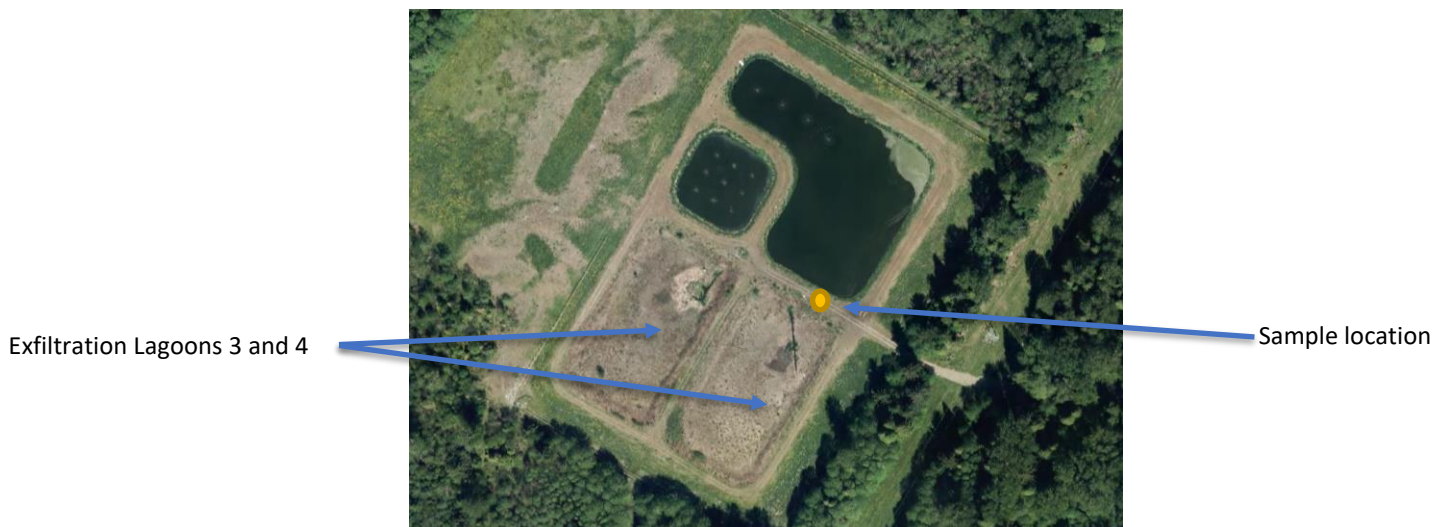
Photo 1. Overview of Queensway Sewer Treatment Facility
