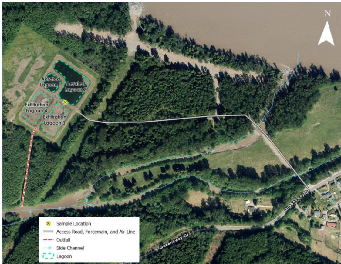
Figure 1 Queensway Sewer Facility, showing the access road and side channels, orthoimagery dated May 2019.
