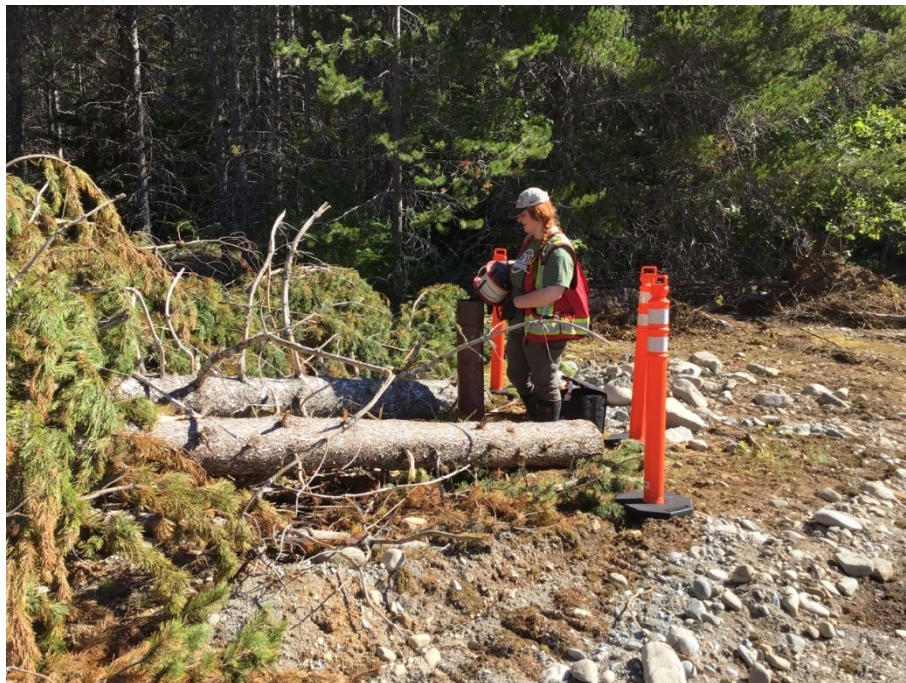
Photo 73: Forceman Ridge Waste Management Facility MW-14, well head, July 27, 2022
