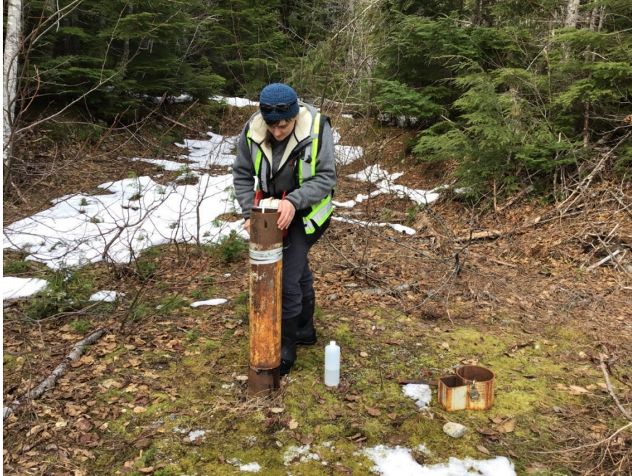
Photo 68: Forceman Ridge Waste Management Facility MW-13, well head, March 25, 2022
