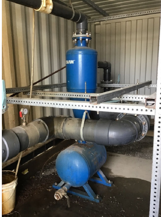
Photo 84: Forceman Ridge Waste Management Facility Sand Filter, August 31, 2022
