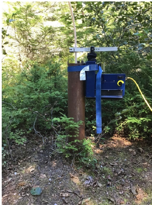
Photo 31: Forceman Ridge Waste Management Facility MW-02, well head, September 1, 2022
