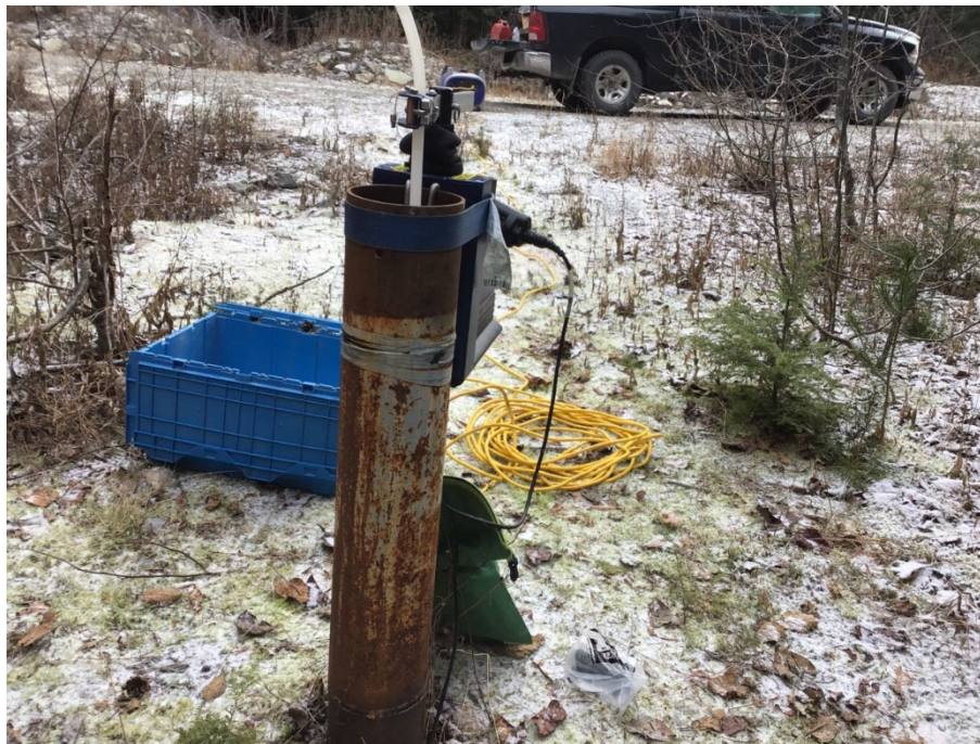
Photo 71: Forceman Ridge Waste Management Facility MW-13, well head, November 30, 2022
