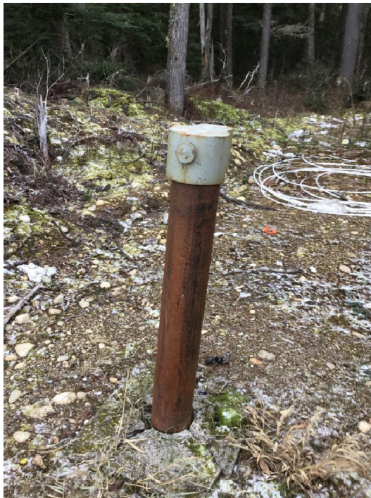
Photo 83: Forceman Ridge Waste Management Facility MW-16, well head, December 1, 2022
