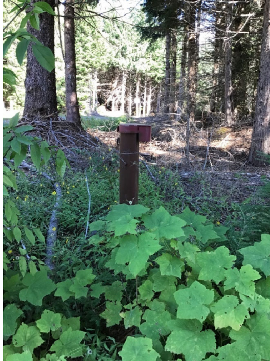
Photo 40: Forceman Ridge Waste Management Facility MW-05, well head, August 31, 2022
