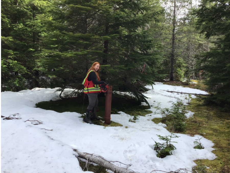
Photo 58: Forceman Ridge Waste Management Facility MW-10, well head, March 25, 2022
