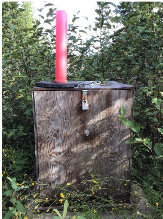
Photo 33: Forceman Ridge Waste Management Facility MW-03, well in wooden casing, August 30, 2022
