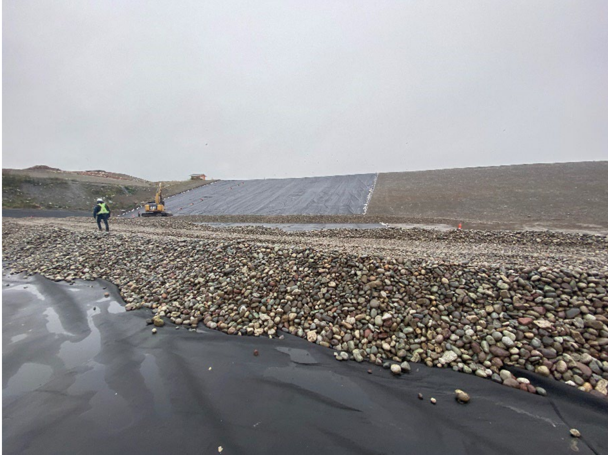
Figure 7: Construction of Cell 1B
