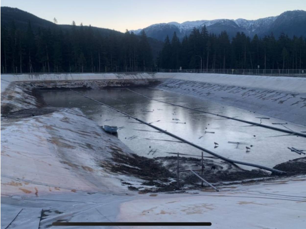
Figure 5: Aeration Pond After Dewatering, October 19, 2022
