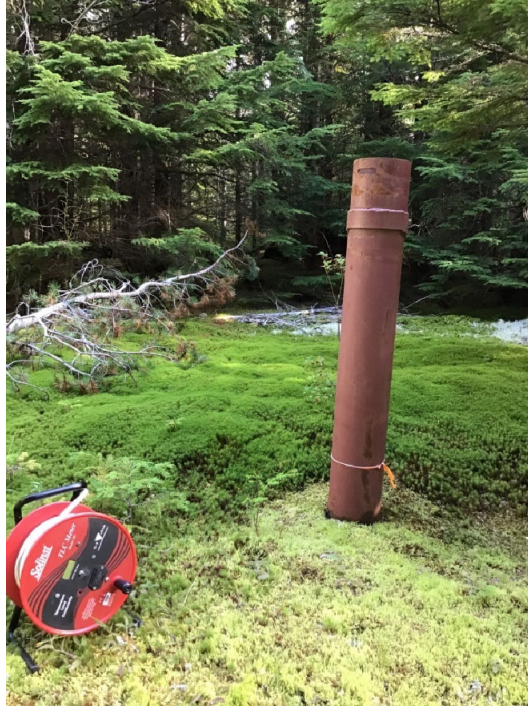
Photo 60: Forceman Ridge Waste Management Facility MW-10, well head, September 1, 2022
