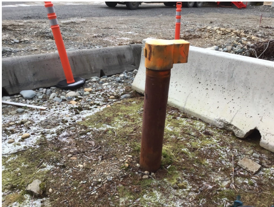
Photo 75: Forceman Ridge Waste Management Facility MW-14, well head, December 1, 2022
