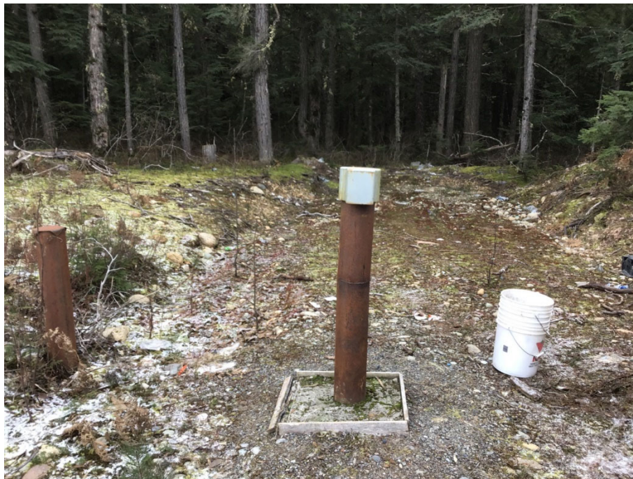
Photo 79: Forceman Ridge Waste Management Facility MW-15, well head, December 1, 2022
