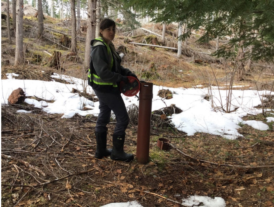
Photo 54: Forceman Ridge Waste Management Facility MW-09, well head, March 25, 2022
