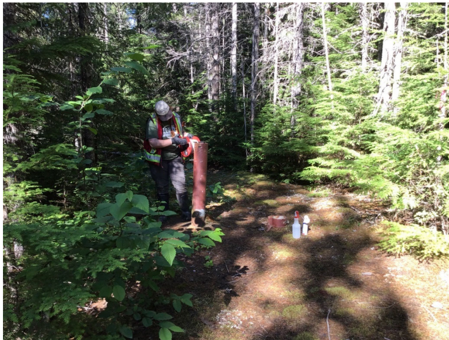
Photo 63: Forceman Ridge Waste Management Facility MW-11, well head, July 27, 2022
