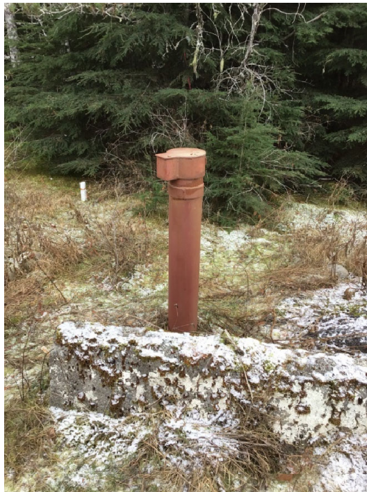
Photo 53: Forceman Ridge Waste Management Facility MW-08, well head, December 1, 2022
