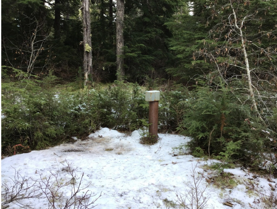
Photo 32: Forceman Ridge Waste Management Facility MW-02, well head, November 30, 2022
