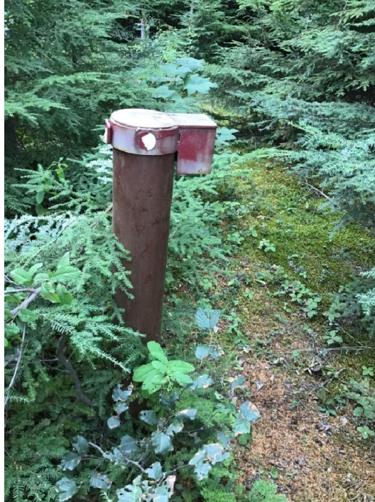
Photo 44: Forceman Ridge Waste Management Facility MW-06, well head, September 1, 2022
