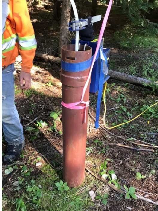
Photo 56: Forceman Ridge Waste Management Facility MW-09, well head, August 31, 2022
