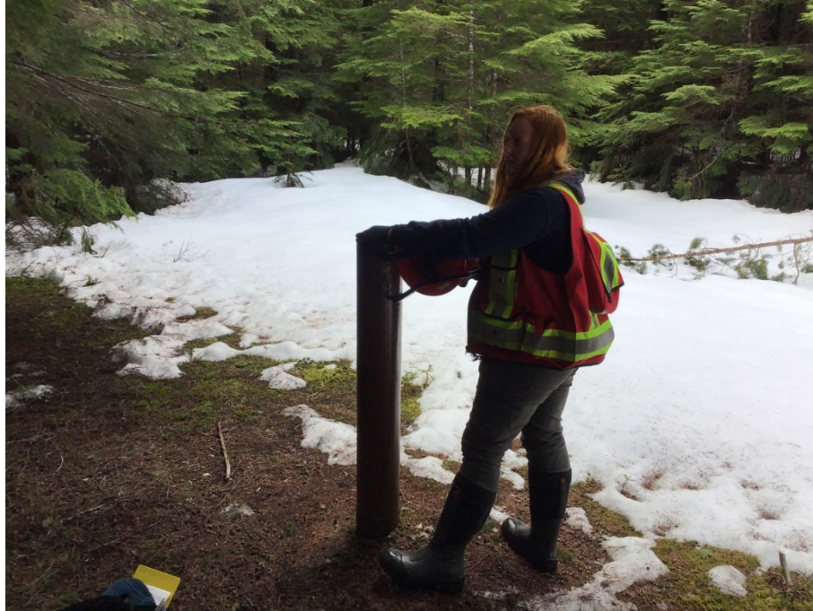
Photo 34: Forceman Ridge Waste Management Facility MW-04, well head, March 25, 2022
