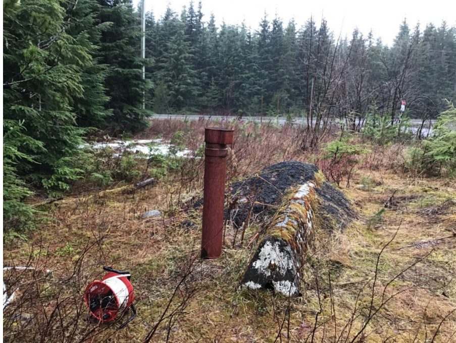
Photo 50: Forceman Ridge Waste Management Facility MW-08, well head, March 25, 2022
