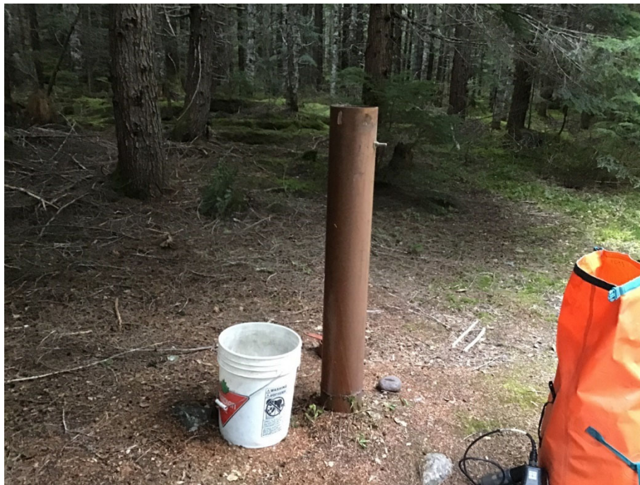
Photo 37: Forceman Ridge Waste Management Facility MW-04, well head, November 30, 2022
