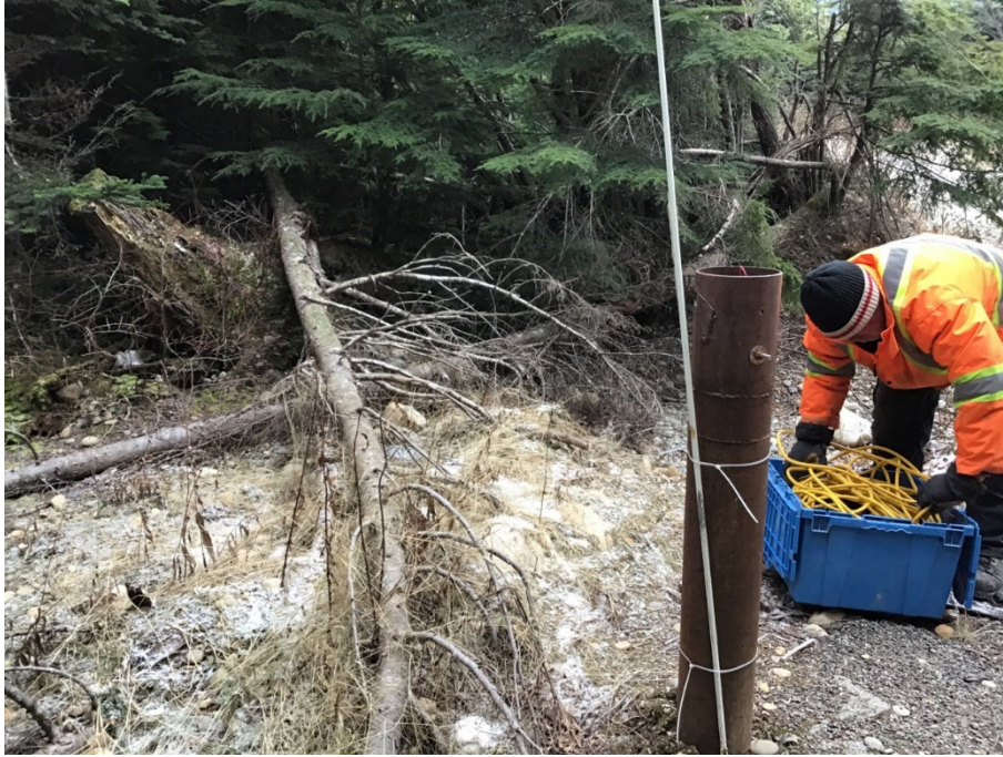
Photo 28: Forceman Ridge Waste Management Facility MW-01, well head, September 1, 2022
