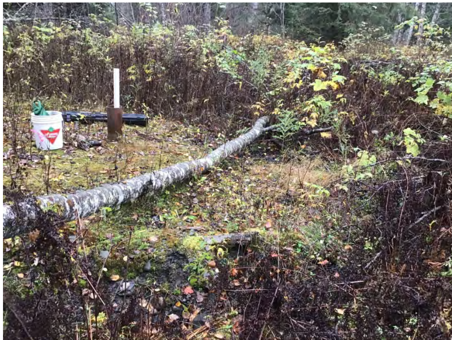
Photo 39: Hazelton Waste Management Facility SGW-05, well, October 18, 2022
