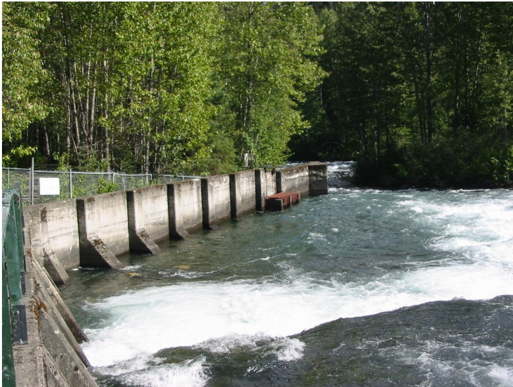
Buttressed concrete side wall of the fish ladder August 2010
