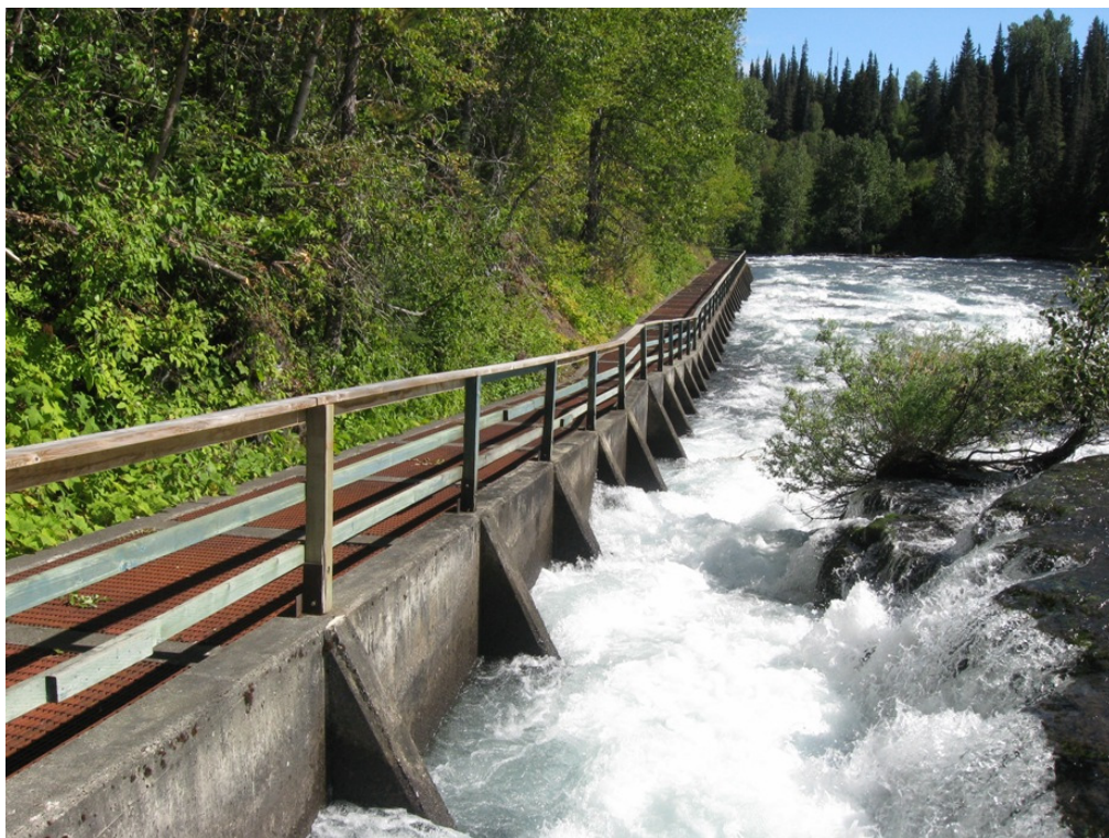
View of walkway, buttressed concrete wall and upper Meziadin Falls looking downriver. August 2010
